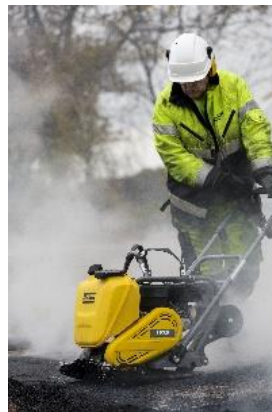
An Atlas Copco plate compactor
