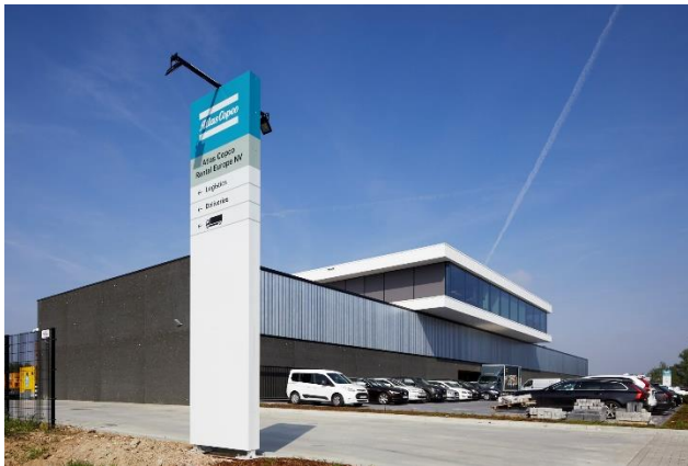
The new facility in Boom, Belgium
