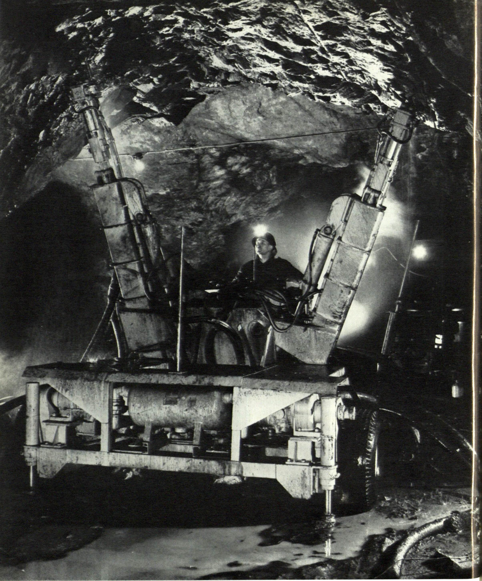
A new technique to mechanize long-hole drilling in mines—the MLD-method—has been introduced by Atlas Copco on an international scale. During its development in Swedish mines it has increased the footage drilled per man-shift by three to five times. The picture shows a Simba rig, basis of the method, in use at Kiruna, Sweden.
