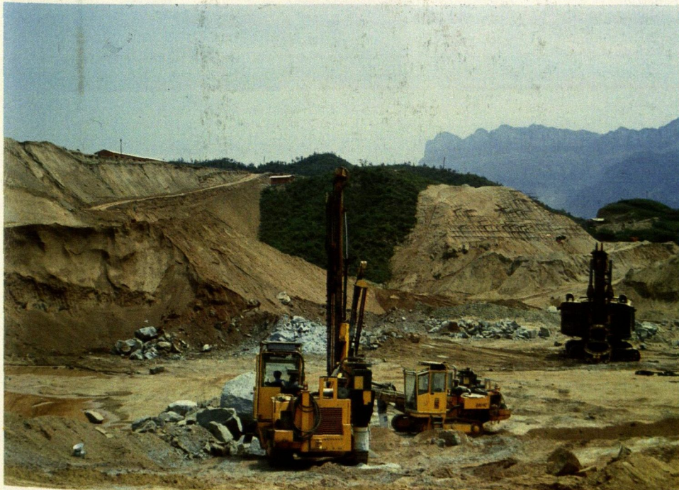
Construction of the Three Gorges power plant project started in 1994 with a large number of Atlas Copco rock drilling rigs.
