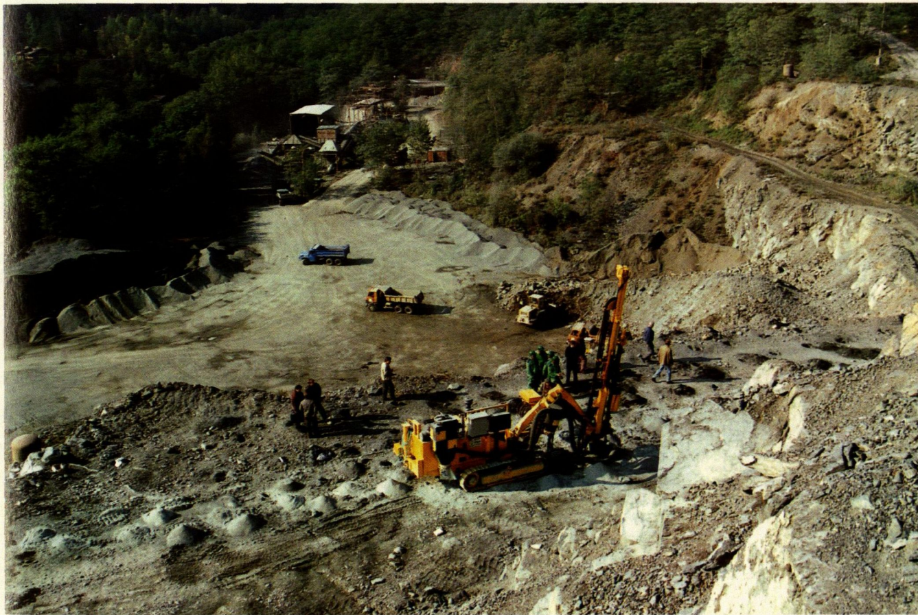
A hydraulic drilling rig in operation at a quarry in the Czech Republic.
