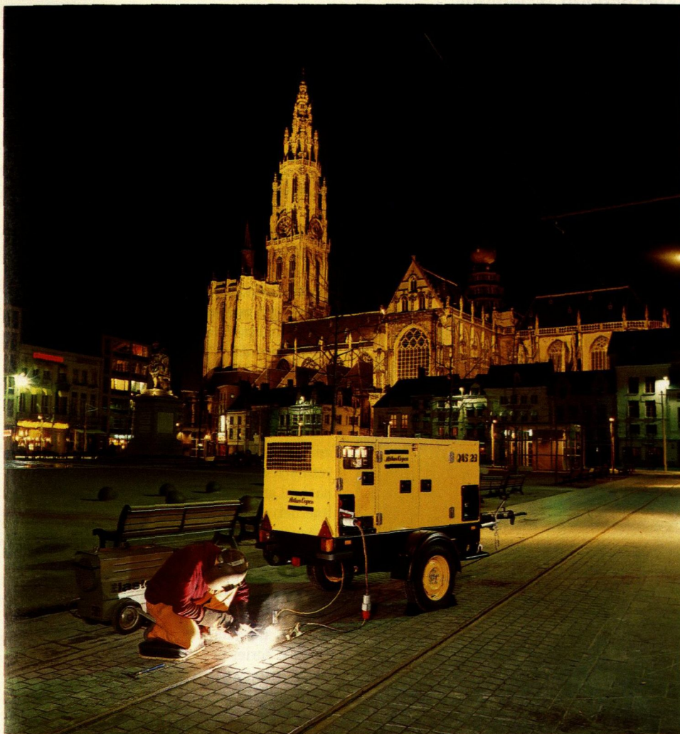
An Atlas Copco generator, used for the welding of tram rails in Antwerp, Belgium.
