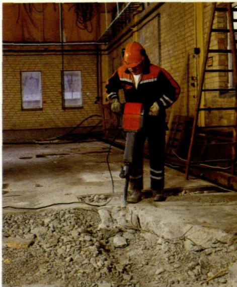
Demolition using an electrically powered Kango breaker.
