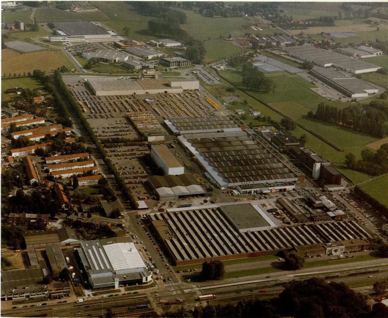
The Compressor Technique industrial complex in Antwerp includes a manufacturing unit for compressor components and three compressor assembly plants.
