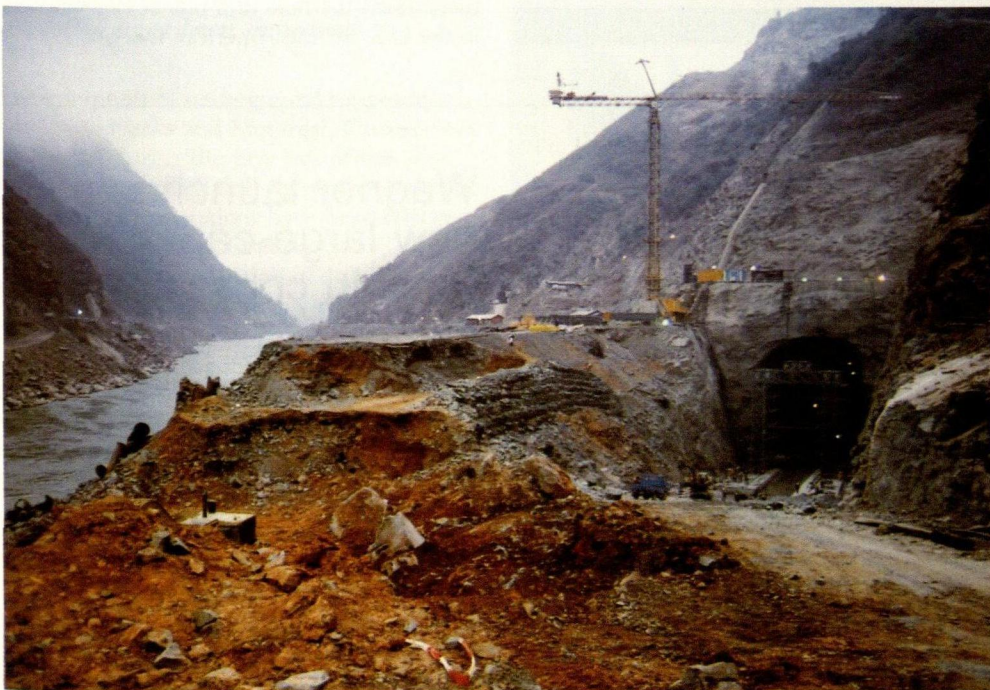
Construction work at Ertan's hydro power plant in China.
