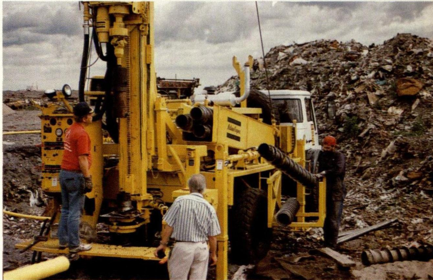
Environmental drilling at the Gladökvärn refuse plant outside Stockholm.
