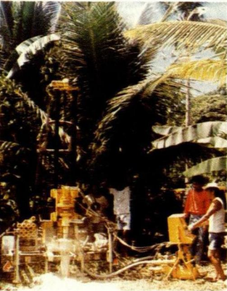
Well-drilling in the Philippines using Aquadrill 60.
