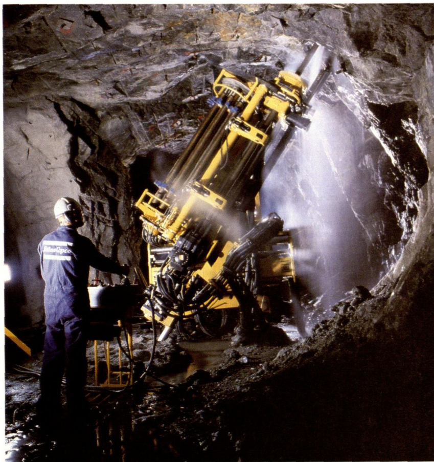
Drilling rig for sub-level caving.
