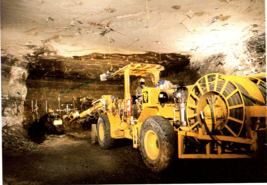
A drilling rig for drifting operations, equipped with the newly developed lightweight hydraulic boom.
