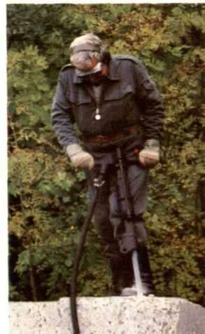
A compressed-air breaker in use with the Swiss Civil Defense Force.
