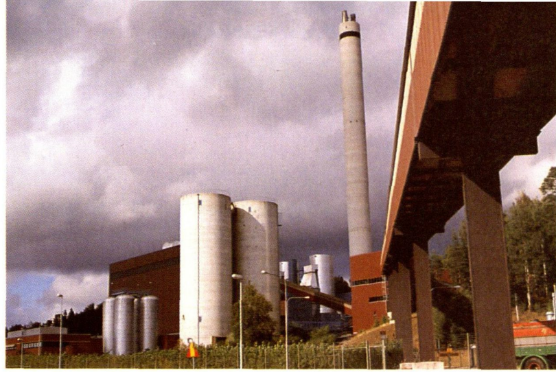
The Igelsta thermal power plant in Södertälje, south of Stockholm.
