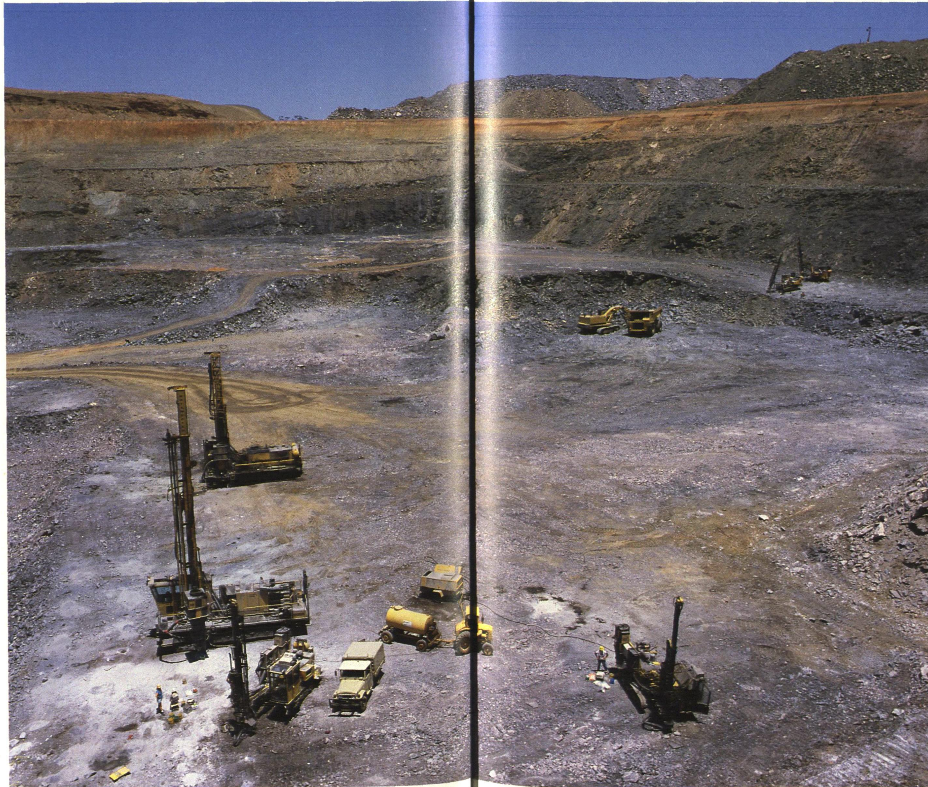
During the past two years, Atlas Copco has sold more than 50 drilling rigs to contractors at gold mines in Kalgoorlie, Australia.
