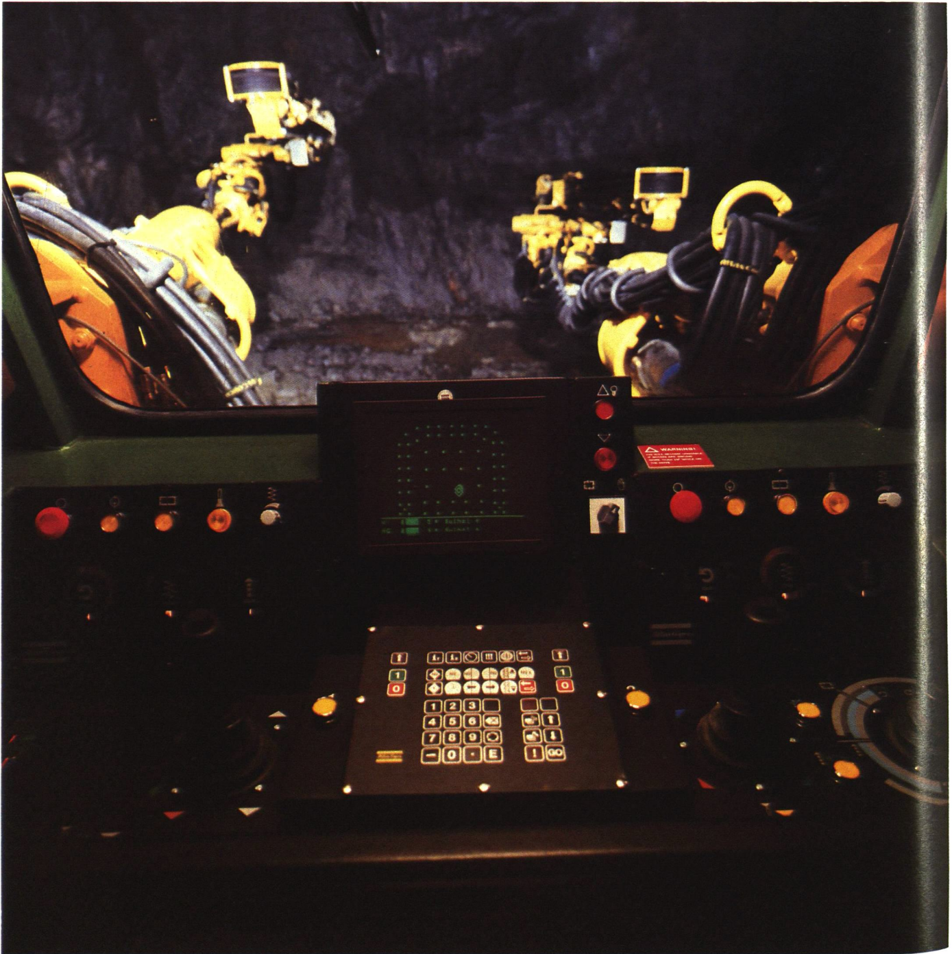
Today, advanced electronics are an integral part of many Atlas Copco products and systems. Examples are painting robots, assembly and automation systems, compressor monitoring and automatic rock drilling rigs. Shown is the interior of a control cab for a fully automatic hole drilling rig which can bore the complete blast hole pattern without operator assistance.
