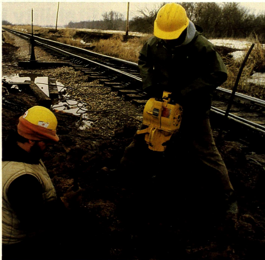
The "Pionjär" gasoline-powered portable combination machine is used for rock drilling, breaking, tamping of cross-ties, digging, etc. This machine is being used to excavate a cable bed along a railroad right-of-way in the U.S.
