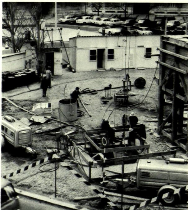
Portable compressors supply air power for tunnelling work in Lisbon—part of the city's flood control measures.
