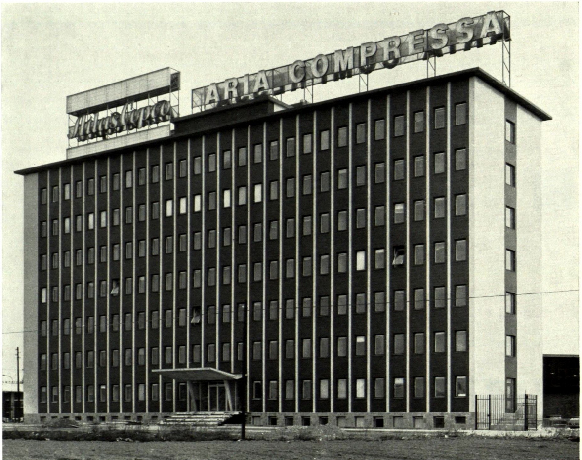
New Atlas Copco premises erected during the year in several countries include this new office building in Milan for Atlas Copco Italia.
