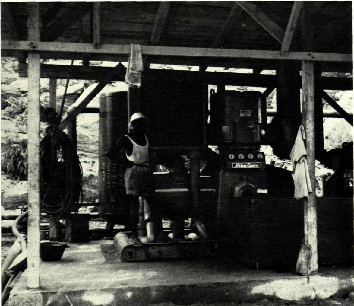
Above: Supplying air power to work for hydro power at Akosombo, site of the main dam in Ghana's Volta River Project. Eight of these ET6 compressors are included in the Company's equipment used by the Italian contractors Impregilo.
