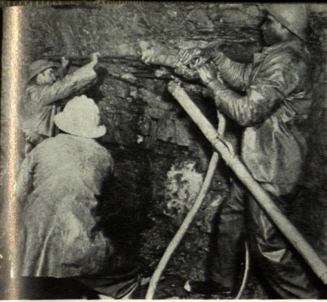
Driving the mile long "Inner Loop" drainage system 60 feet below the heart of Rochester, New York, using "Lion" rock drills with Sandvik Coromant drill steels.
