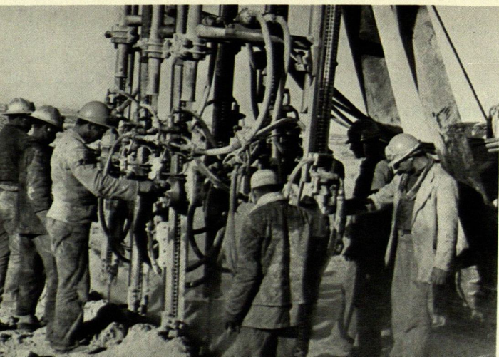
Chain fed rock drills being used in the construction of the oil pipe line Hassi—Messaoud—Bougie in Algeria.
