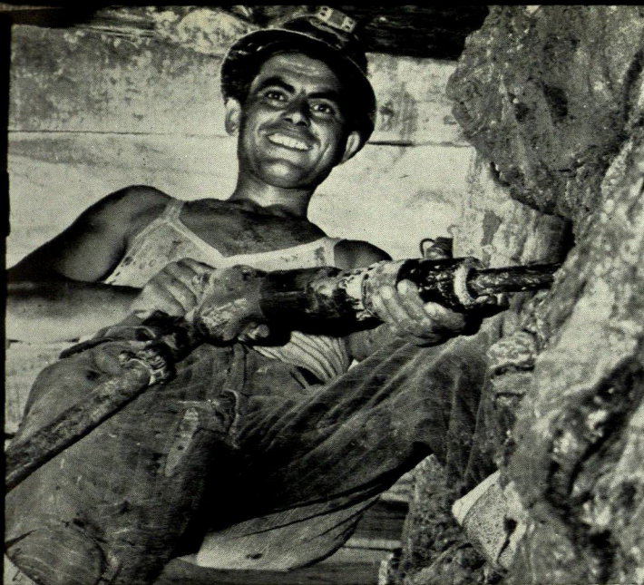
An Atlas Copco clay digger in use during the construction of a tunnel for the Autostrada del Sole in Italy.
