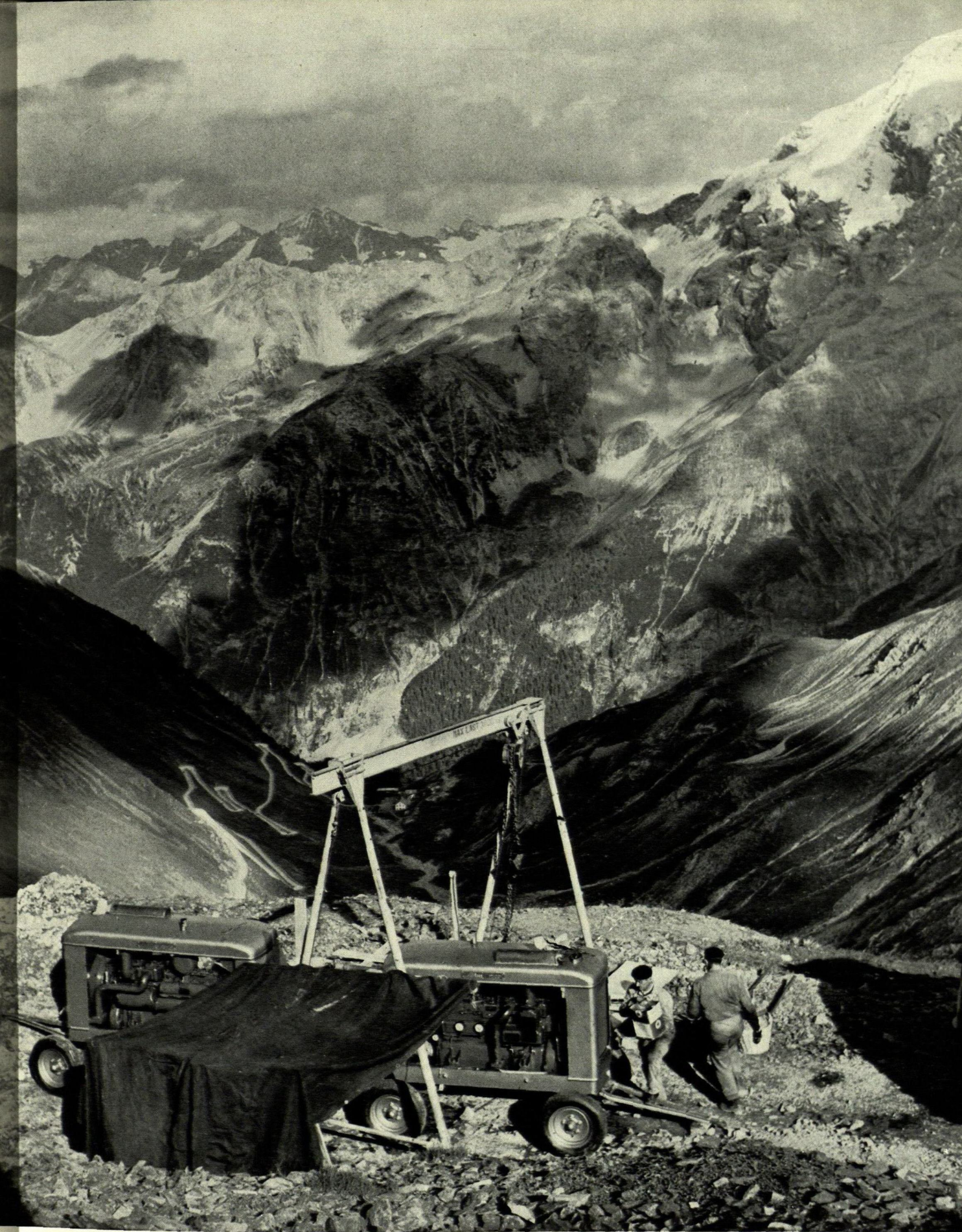
Portable Atlas Copco compressors at work at an altitude of 8,350 ft. on the Stelvio Pass in the Italian Alps.
