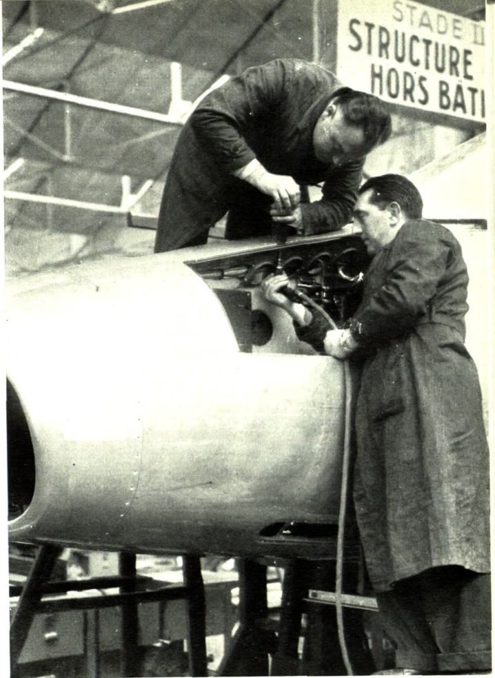
The aircraft industry is one of the branches in which Atlas Copco pneumatic tools are being increasingly used. Here we see an Atlas Copco riveting hammer being used during the manufacture of the French Super Mystère jet fighter.
