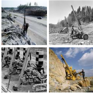
Pneumatic drill rigs 1960-2004
