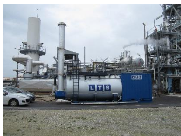
An LTS steam boiler
