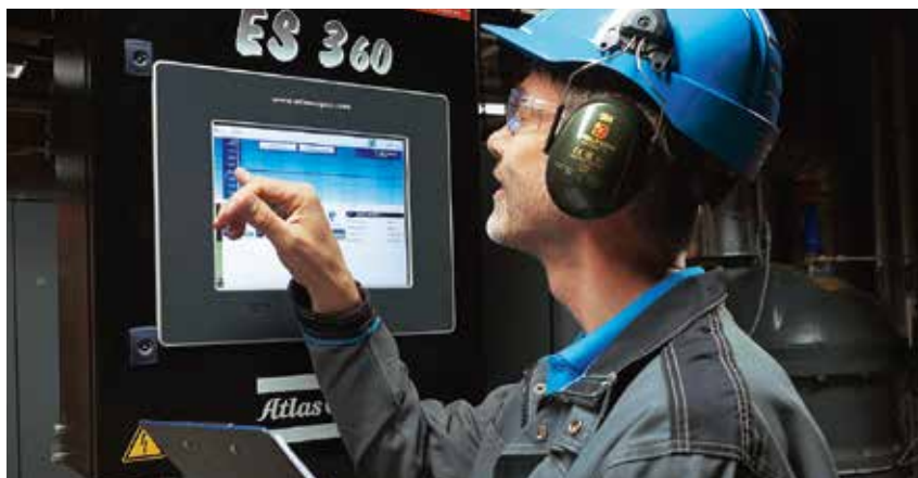
About the image: Efficient compressor management is a fast way to achieve energy savings. Using advanced control systems can save energy. The Atlas Copco ES 360 controller can connect up to 60 machines.
