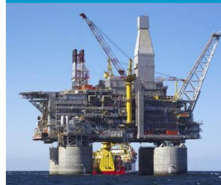
Energy / Oil & gas
